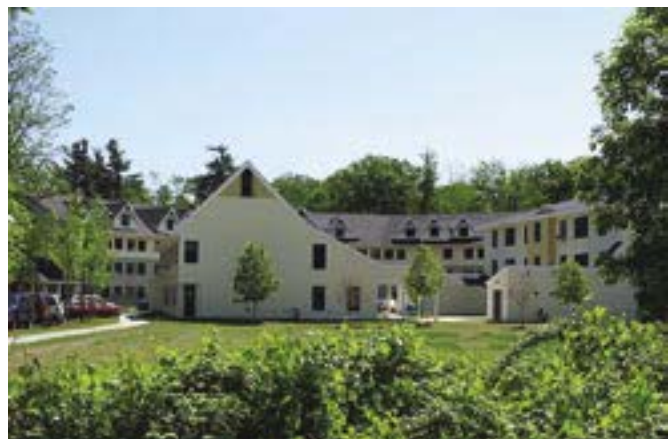
McAuley Square Housing was designed to provide affordable housing for multi-generations with unique special needs.
